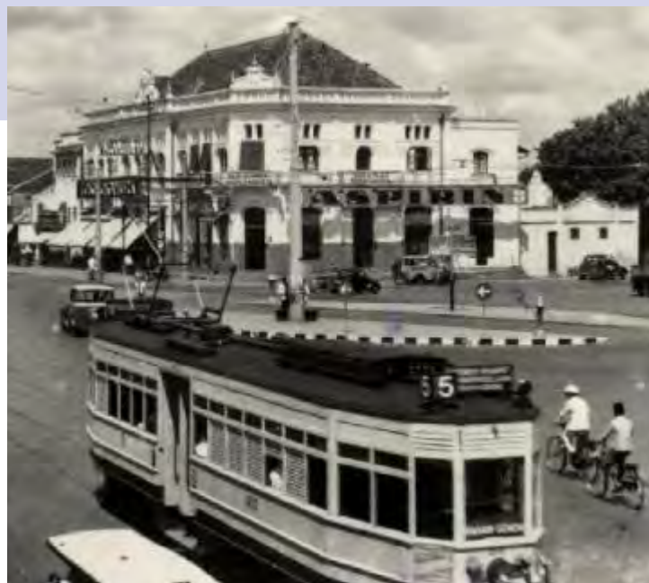
A peaceful-looking street scene in Jakarta during the first year of the Revolution in 1945. The tranquility would not last long.
