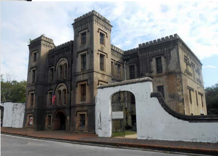
Figure 16. The Old Charleston Jail as it appears
